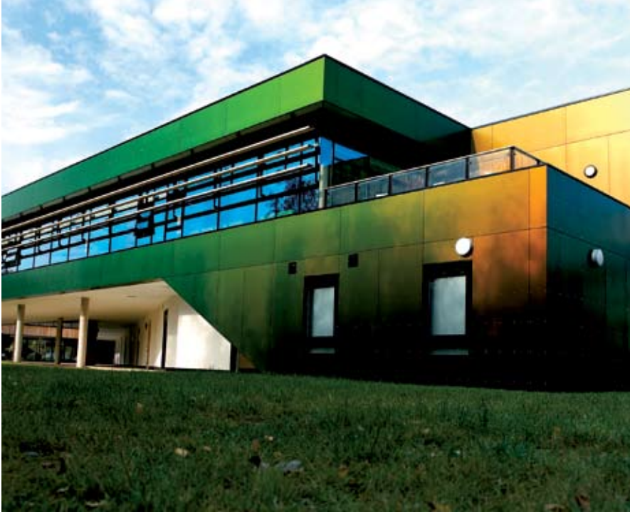
Innovation Centre Lincoln, UK equipped with Rockpanel® chameleon cladding
